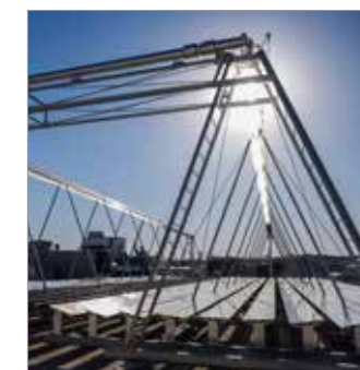
Fig.2 - Linear Fresnel Reflectors at RAM plant in Jordan (source: Industrial Solar)
