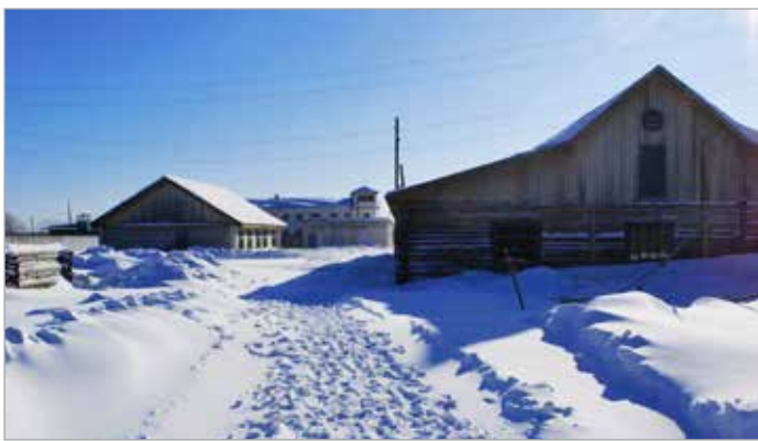
Fig. 1 - Buildings of the Perm-36 Memorial Museum of the History of Political Repression and Totalitarianism. Source: M. Mikaelyan 2018.
