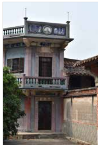
Fig. 1 - One of the abandoned buildings in Dongda village. Reinforced concrete hexagonal turret, which hybridizes the traditional complex
