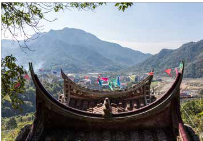
Fig. 1 - The rural settlement assumed as the case study by the dissertation. November 2017
