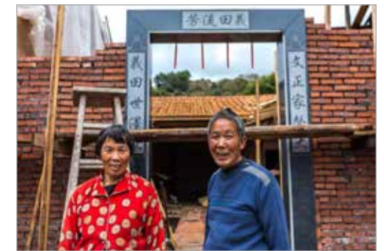
Fig. 3 - Two carpenters are repairing the family temple devoted to their ancestors. December 2018
