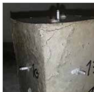
1. Macrocracking in concrete specimen due to the formation of secondary ettringite
