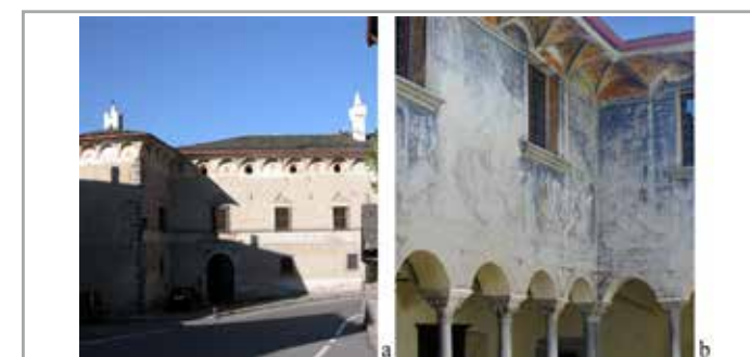
Fig.3 - Palazzo Besta (a) and detail of the treated painted plasters (b).
