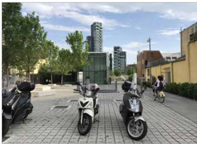
Fig. 1 - Permeable pavement installed at Gaetano di Castiglia street, Milan (Italy).
