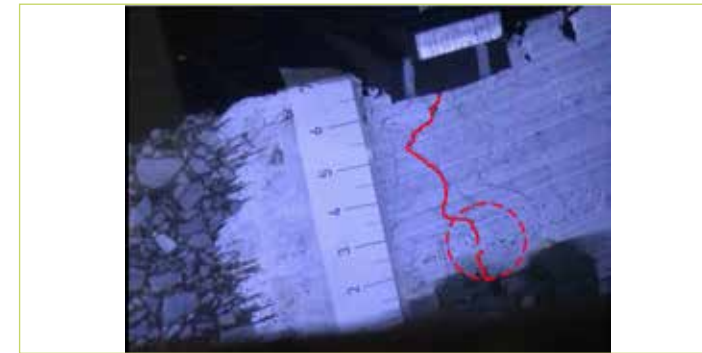
2. Crack path in unreinforced double-layered system.
