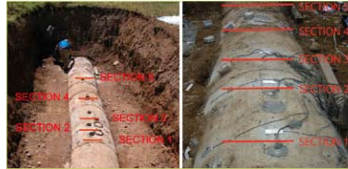
2. Blast tests set-up on the embedded concrete pipe
