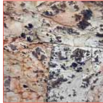
2. Calcium oxalate films on red limestone on the exterior stone lining of the Arena in Verona
