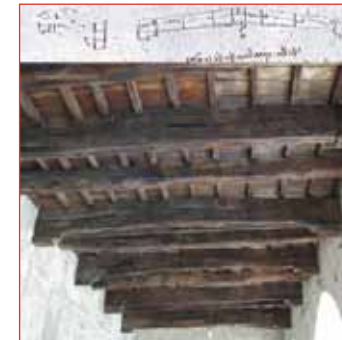
1. Sketch by Leonardo da Vinci's "Codice Atlantico" of a three pieces composite beam and, below, similar beams in the castle of Pandino (XIV century)
