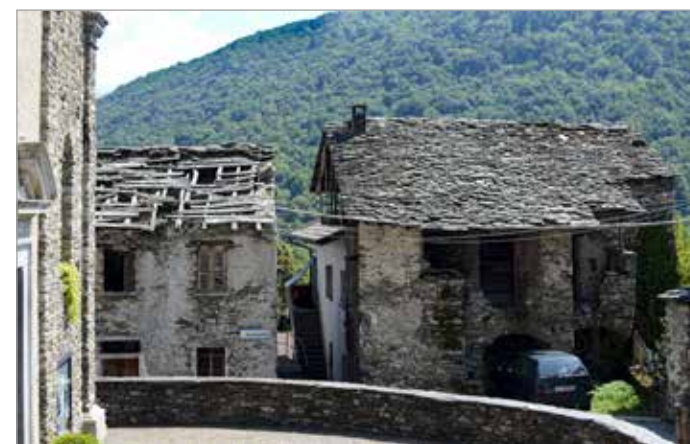
Fig. 3 - Buildings in a state of ruin in the ancient part of the settlement of Livo (CO). The abandonment involved the collapse of the roofs and the perimeter walls (photo taken in 2018)
