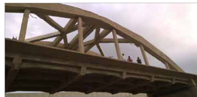
Fig. 2 - The reinforced concrete bridge built in 1935 in the lowland near Sabarguma (Nelly Cattaneo 2018)
