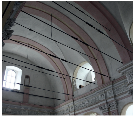
3. Santa Casa Lauretana, Tresivio (Northern Italy). Tie-rods contrasting the thrusts of the masonry vaulted structure to be understood and preserved.
