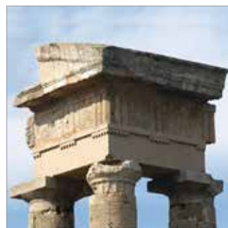
2. Acropolis of Rhodes (Greece), Temple of Pythian Apollo. Detail of the entablature reassembled between 1938-1940 by Italian Archaeological mission with the aid of reinforced concrete.
