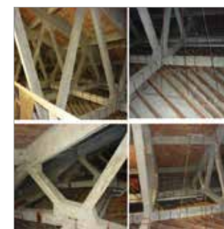
2. Roof trusses designed by Luigi Santarella
