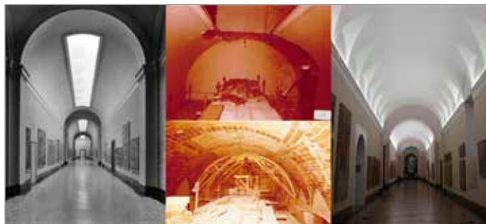
1. Pinacoteca di Brera, room 1, the 50's vaulted ceiling designed by architect Piero Portaluppi and the current one after the 70's stylistic re-composition. Courtesyarchivio fotografico Soprintendenza beni storico artistici and Soprintendenza beni architettonici, Milano.
