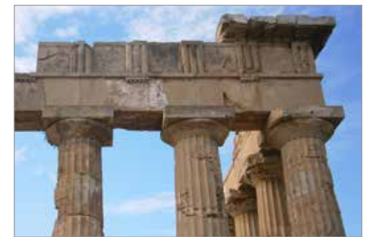
1. Selinunte (Sicily), Temple E, detail of a colonnade reassembled between 1956-1959 with the aid of reinforced concrete under the direction of archaeologist Iole Bovio Marconi.
