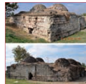
3. 15 th century historical structure (GaziMihalBey Bath, 1421 A.D.) in Edirne-Turkey. The corners of the building constructed with materials more durable, which was done in purpose for keeping the structure more stable for horizontal loads. On the upper photograph, strengthened corner of the building was seen. On the lower photograph, collapsed corner was seen.
