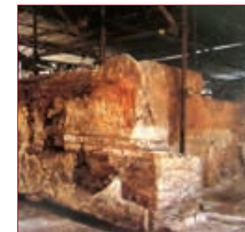
1. Rimini, surgeon's Domus, earth wall on brick footing.
