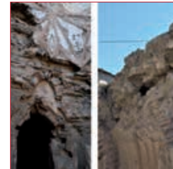
2. 15 th century historical structure (Ismail Bey Bath) in Iznik-Turkey. Timber tie beam holes were located inside the walls of the structure. Timber tie beams were kept together the masonry walls for the horizontal loads.
