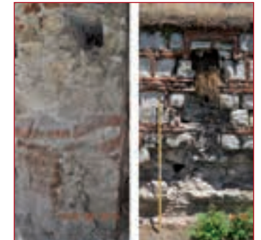
4. 15 th century historical structure (GaziMihalBey Bath, 1421 A.D.) in Edirne-Turkey. The timber tie beam holes were inside of the masonry structure. As well the brick knitting patterns were behave like a horizontal beam around the perimeter of the structure against the horizontal loads.
