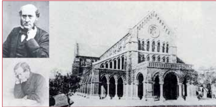
1. The first high form of duotone brickwork architecture, Holy Trinity Church at Shanghai, 1869, by Sir Gilbert Scott (1811-1878) and William Kidner (1844-1900). (the photograph of the architecture in: Chen, Congzhou, Zhang, Ming (eds), Shanghai jindai jianzhushi gao , 1988, p.89)
