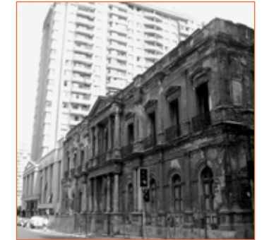
2. The decay of the Chilean architectural heritage. Palacio Pereira, Santiago de Chile (Photograph taken by Maria Victoria de los Angeles Correa Baeriswyl)
