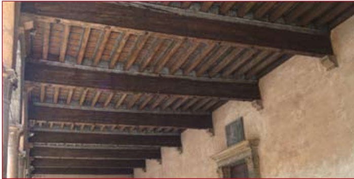
2. Composite beams in Council's Loggia, Verona (XV th century)
