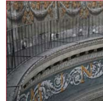
2. S. Andrea Basilica, Mantua. A circular pipe, which supplied 250 small gas burners, is still preserved at the base of the tambour
