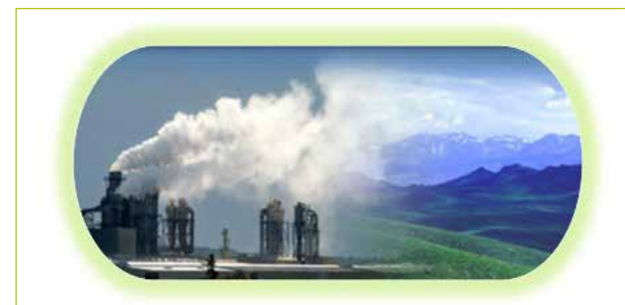
1. Acid gas removal by amine scrubbing is widely used to control the composition of gaseous streams leaving process plants
