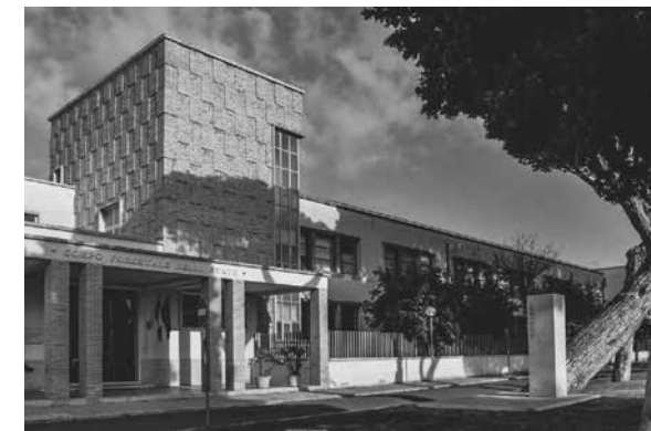
Fig. 2 Author's photographic survey 2018. Elementary school in Sabaudia by Oriolo Frezzotti (1934)
