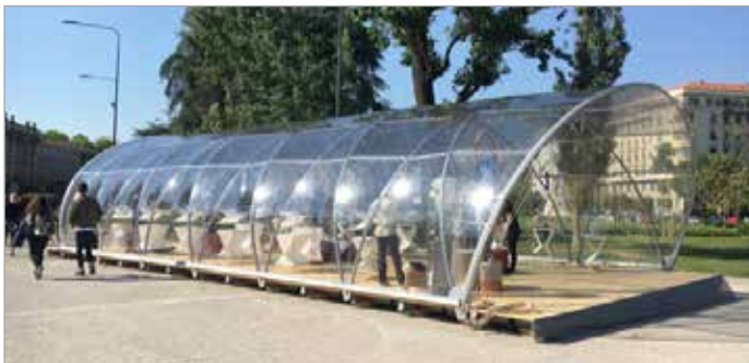
Fig. 1 - Pilot project “TemporActive” (a hybrid bending active ultra-lightweight temporary structure), developed as experimental part of the doctoral thesis.
