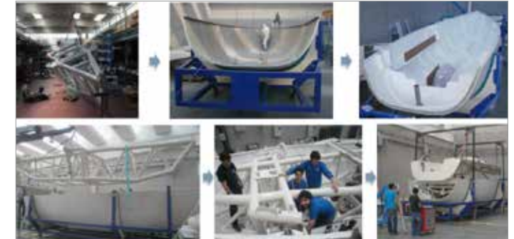
Fig.1 Sailing Yacht Laboratory Building Process: Dynamometric Test Rig.
